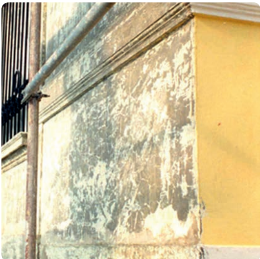
Façade after paint removal
